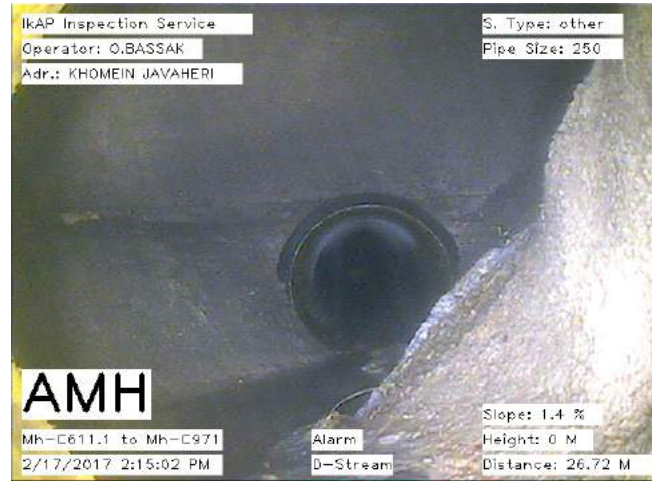
Photo : 5.jpg 26.72 m, Manhole # 6
